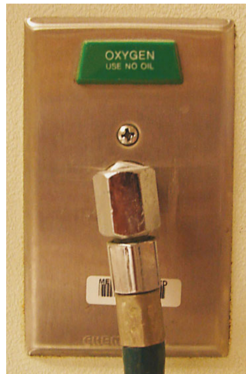
Figure 1-6. Wall oxygen source, which is color-coded green (in the United States) and specifically fitted for oxygen connectors and tubing.
